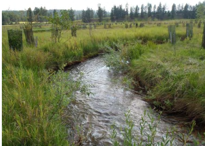
Figure 41. Instream cover provided by willows installed in coir log and willow fascine structures.
